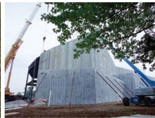
May 9, 2006: Outside wall panels on the north side of the Purser Center are in place.
