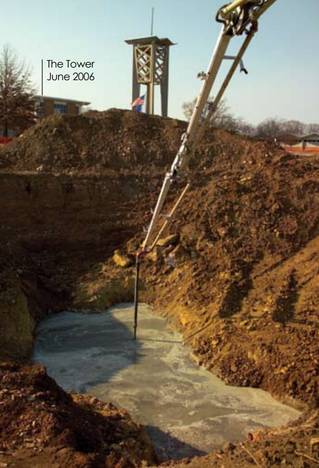
December 7, 2005: More than 80 truckloads of concrete were used to fill the sinkhole at the Purser Center construction site.
