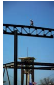
April 10, 2006: Workers on the high beams must remove and replace their safety harnesses after every few feet of movement.
