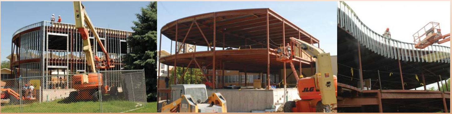
Construction continues on schedule on the new Education Wing building on the Logan campus. The building is expected to be completed in January 2012.
